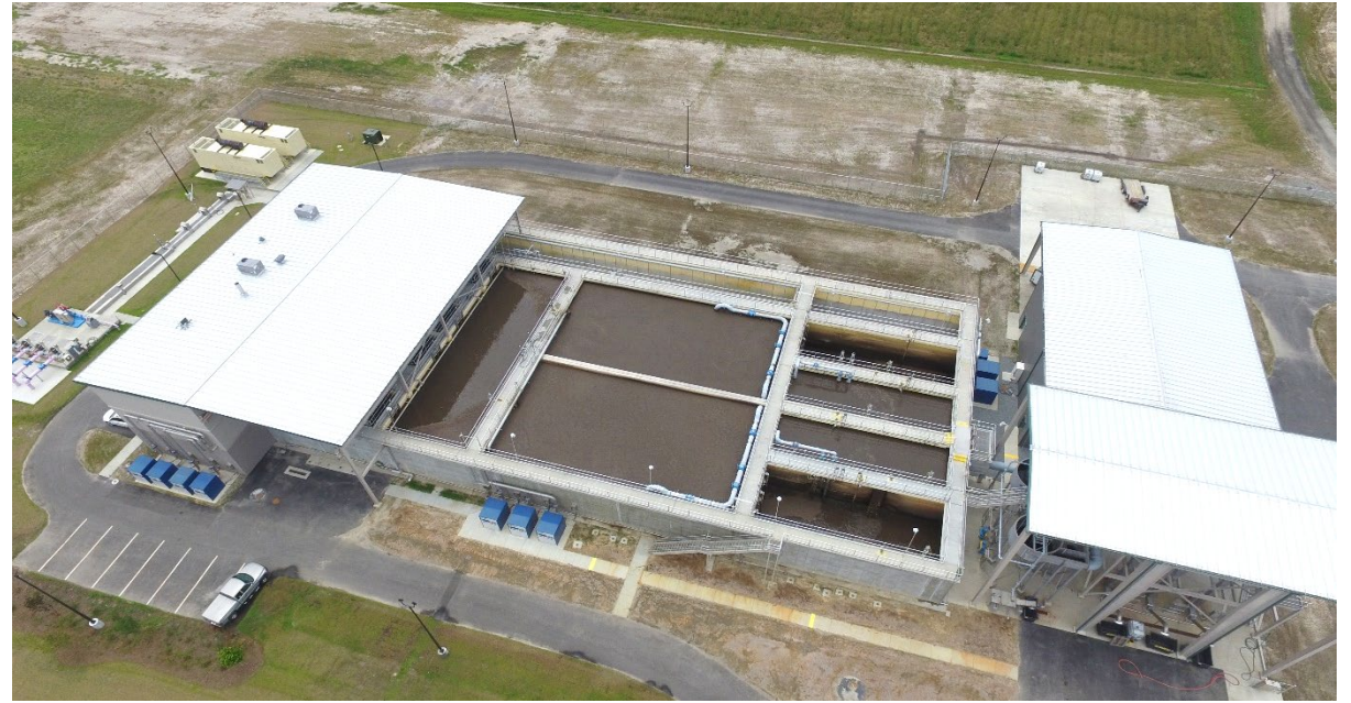
City of Richmond Hill Sterling Creek 4.0 MGD WWTP Richmond Hill, GA Completion Date: 2016 Size: 4.0 MGD flat plate membrane BNR plant
