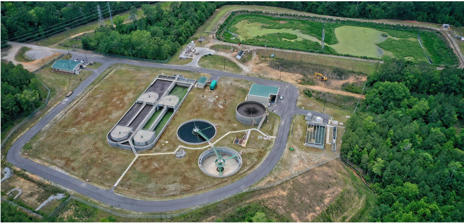
Town of Chapin 2.4 MGD WWTP Chapin, SC Completion Date: 2020 Size: 2.4 MGD oxidation ditch type plant, new construction
