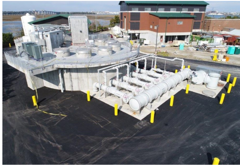
Charleston Water System Phase V West Ashley Sewer Tunnel & Inflow Pump Station Charleston, SC Completion Date: 2022 Size: 120-foot-deep, 1.6-mile-long tunnel and new 60 MGD influent pump station
