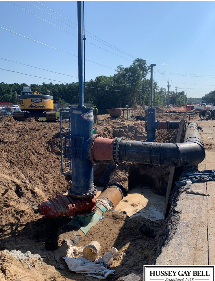
Charleston Water System, Water/Wastewater Utility Relocations for Clements Ferry Road Widening Project Charleston, SC Completion Date: P1 - 2017; P2 - 2024 Size: 30" water main and 24" wastewater force main
