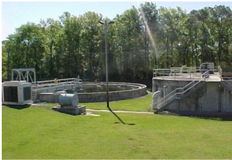
Georgetown Water Reclamation Facility Savannah, GA Completion Date: 1972-2004 (original + multiple expansions) Size: 2.45 MGD oxidation ditch type
