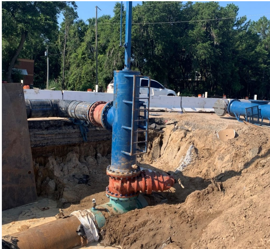
Charleston Water System, Water/Wastewater Utility Relocations for Clements Ferry Road Widening Project Charleston, SC Completion Date: P1 - 2017; P2 - 2024 Size: 30" water main and 24" wastewater force main
