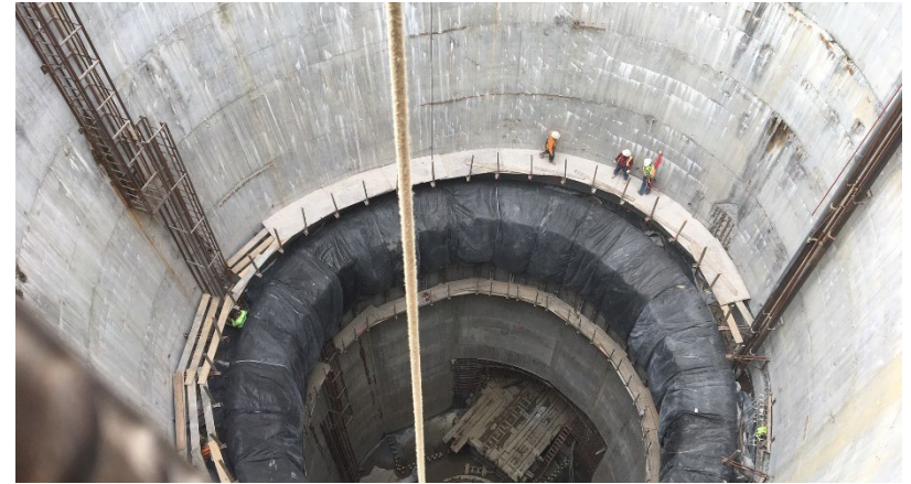
Charleston Water System Phase V West Ashley Sewer Tunnel & Inflow Pump Station Charleston, SC Completion Date: 2022 Size: 120-foot-deep, 1.6-mile-long tunnel and new 60 MGD influent pump station
