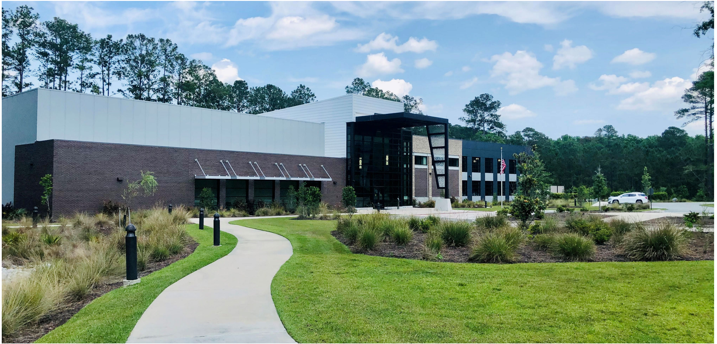
Georgia Advanced Manufacturing Training Center, Quick Start, Pooler, GA Construction Cost: $17.6M Role: Civil engineering
