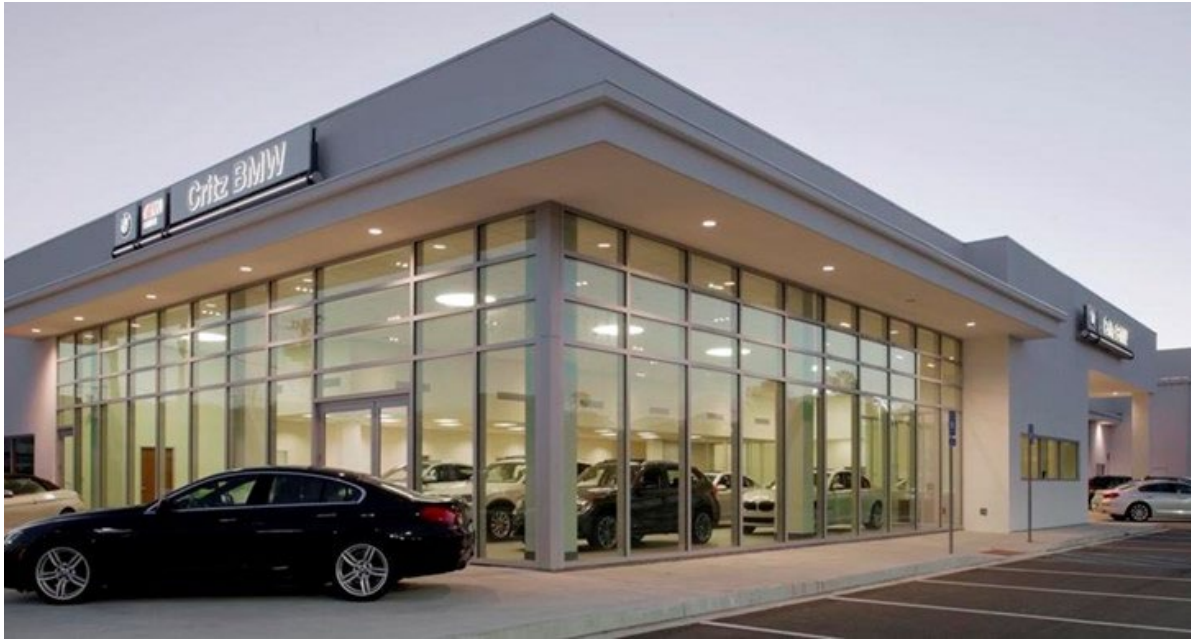
Critz BMW Dealership Savannah, GA Size: 34,700 SF Role: Architect & Engineer of Record
