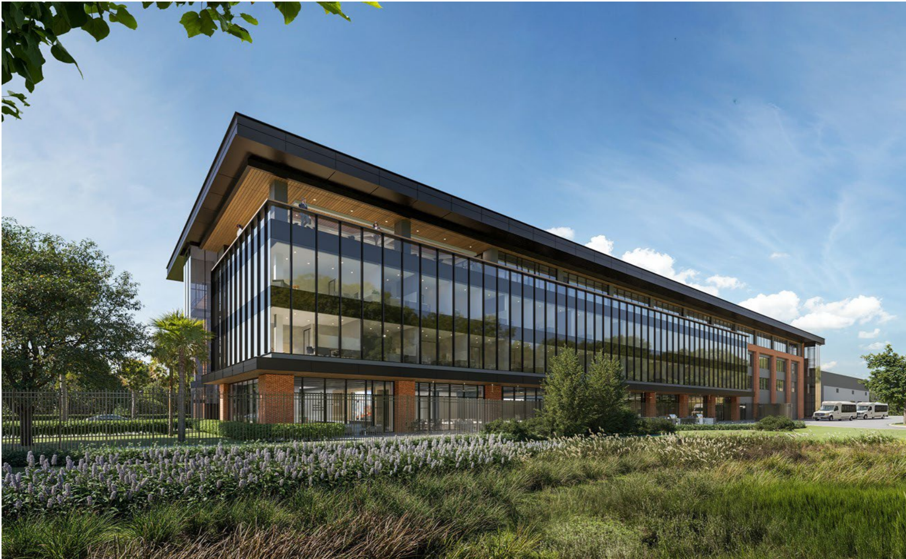
Georgia Ports Authority's Maintenance, Operations & Administration Complex, Garden City Terminal, GA
