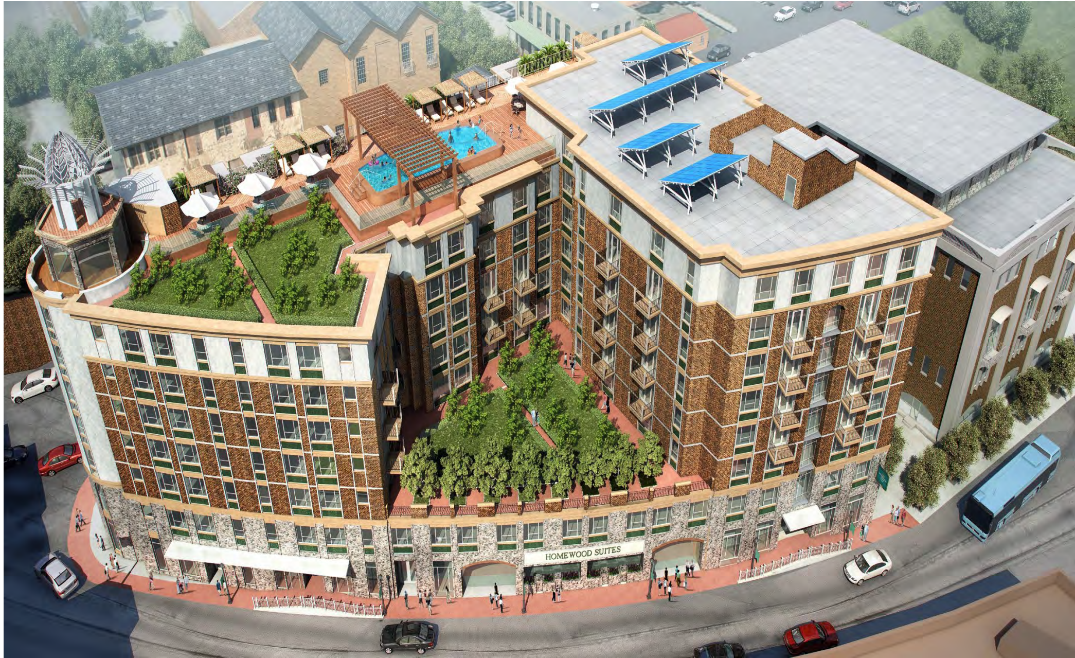
Homewood Suites by Hilton Savannah, GA Size: 162 units Role: Civil Engineering & Site Development
