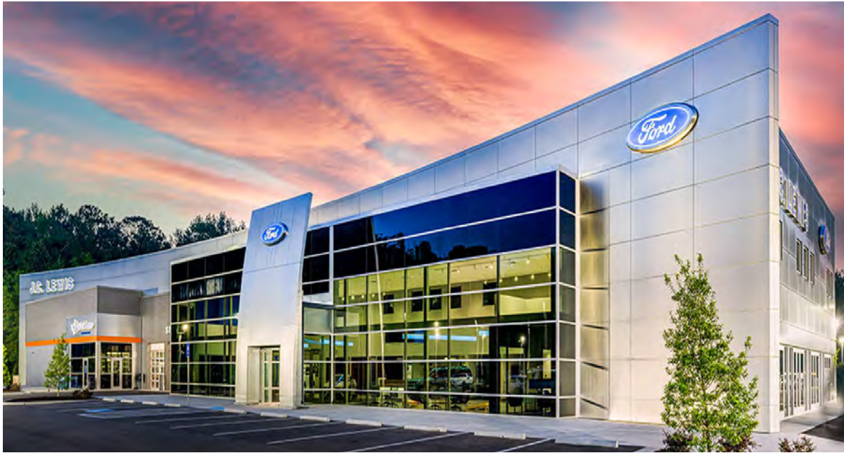
J.C. Lewis Ford Dealership & Quick Lane Service Center, Pooler, GA Size: 54,500 SF Role: Architect & Engineer of Record
