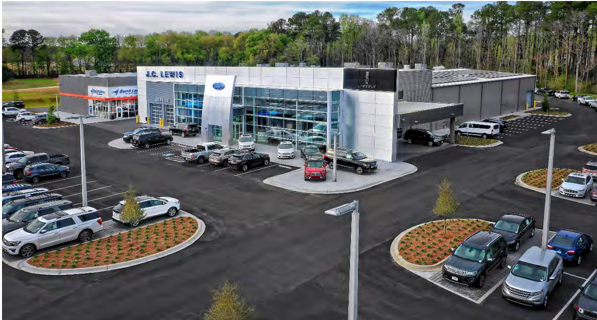
J.C. Lewis Ford Dealership & Service Center Statesboro, GA Size: 30,900 SF Role: Architect & Engineer of Record
