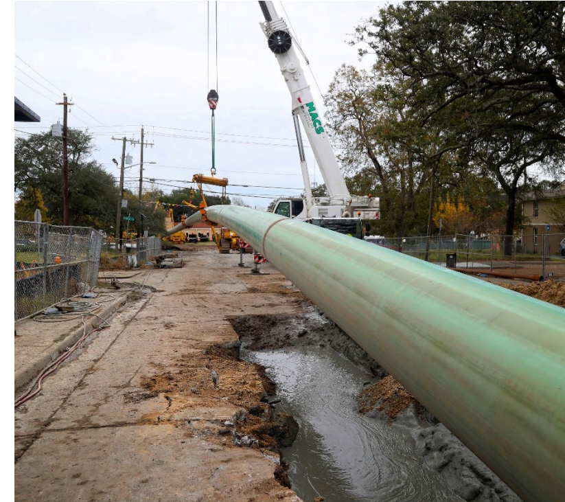
Lift Station 23 Upgrades, Force Main & HDD Savannah, GA Completion Date: 2023 Size: 6,000 LF of 30-inch Fusible PVC
