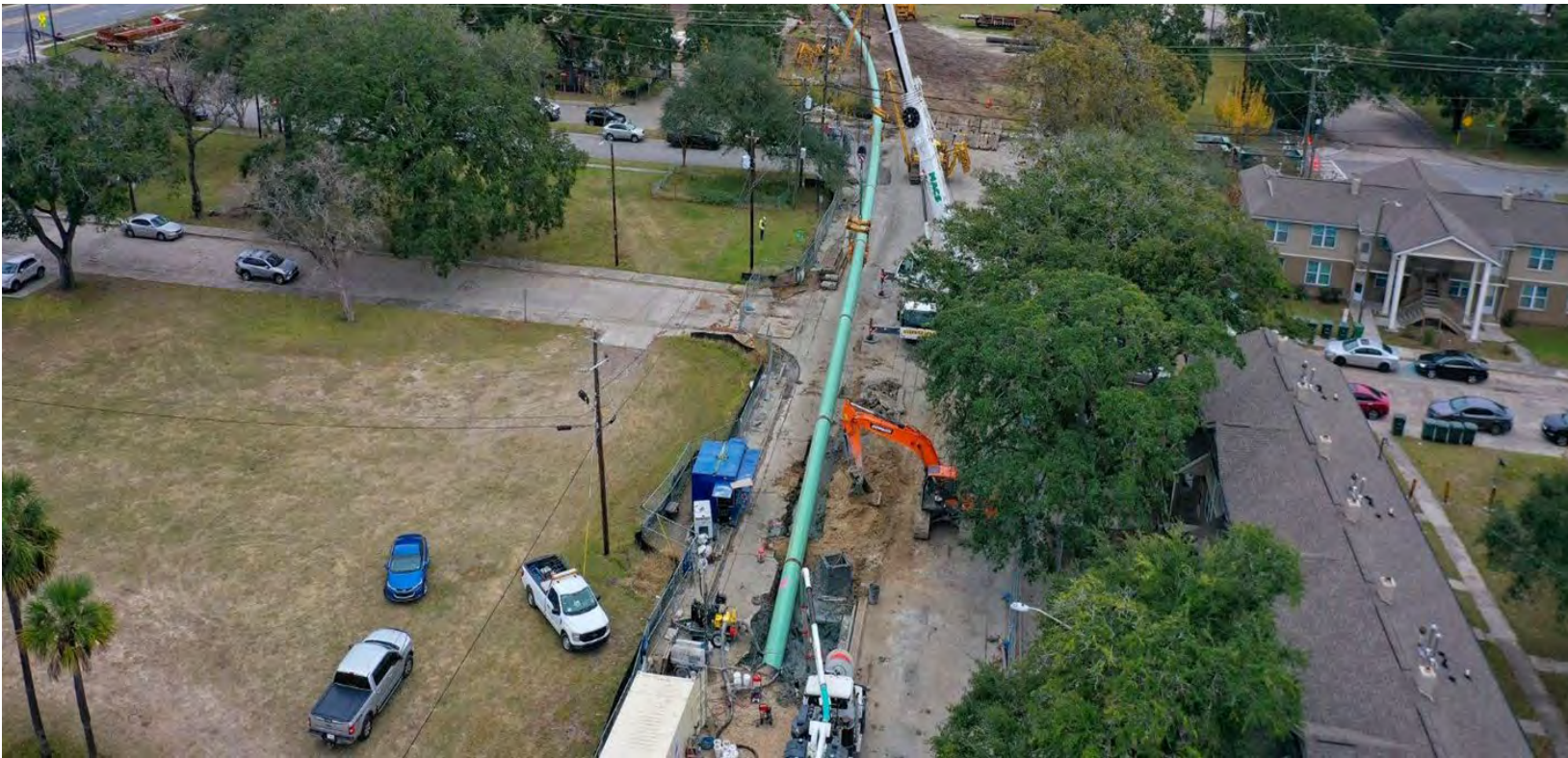
Lift Station 23 Upgrades, Force Main & HDD Savannah, GA Completion Date: 2023 Size: 6,000 LF of 30-inch Fusible PVC
