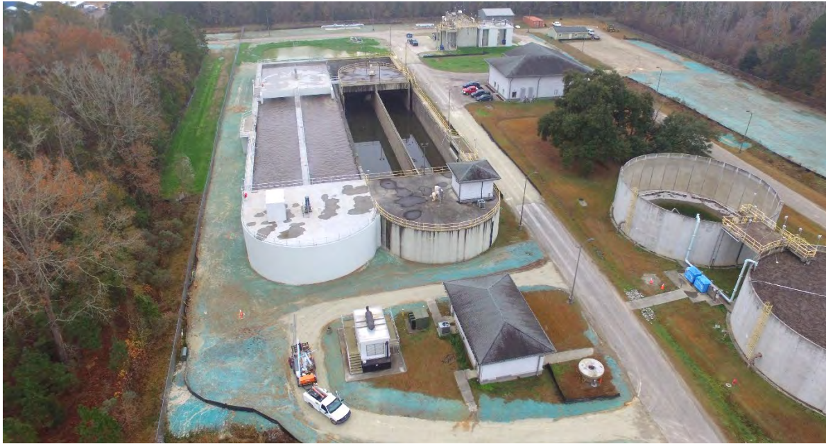
Central Berkeley WWTTP Upgrade to 6.0 MGD Berkeley County, SC Completion Date: 2021 Size: 3.0 MGD expansion of an existing oxidation ditch type plant (upgrade from existing foreign design)
