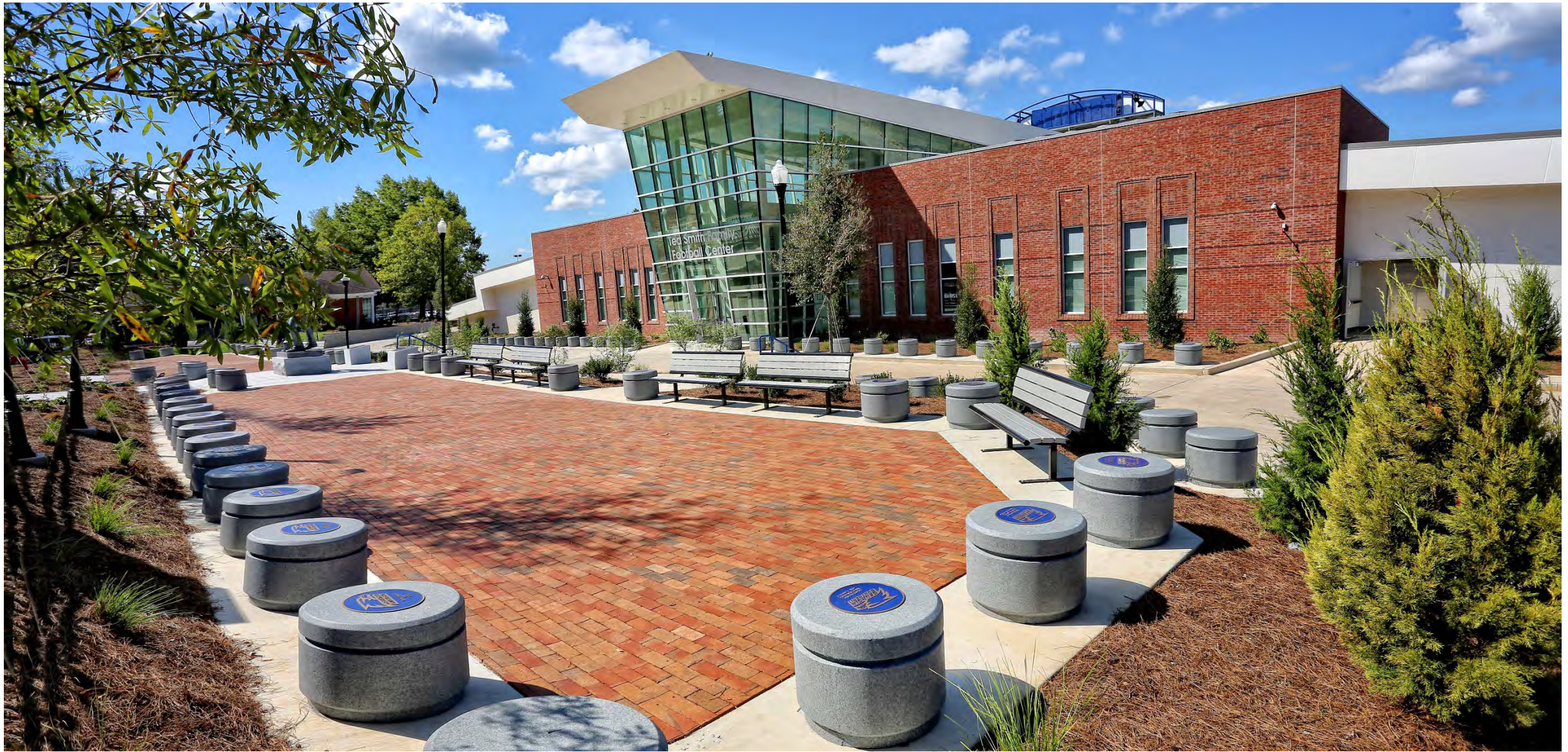
Football Operations Center, Georgia Southern University, Statesboro, GA Size: 57,000 SF Construction Cost: $10M Role: Civil engineering
