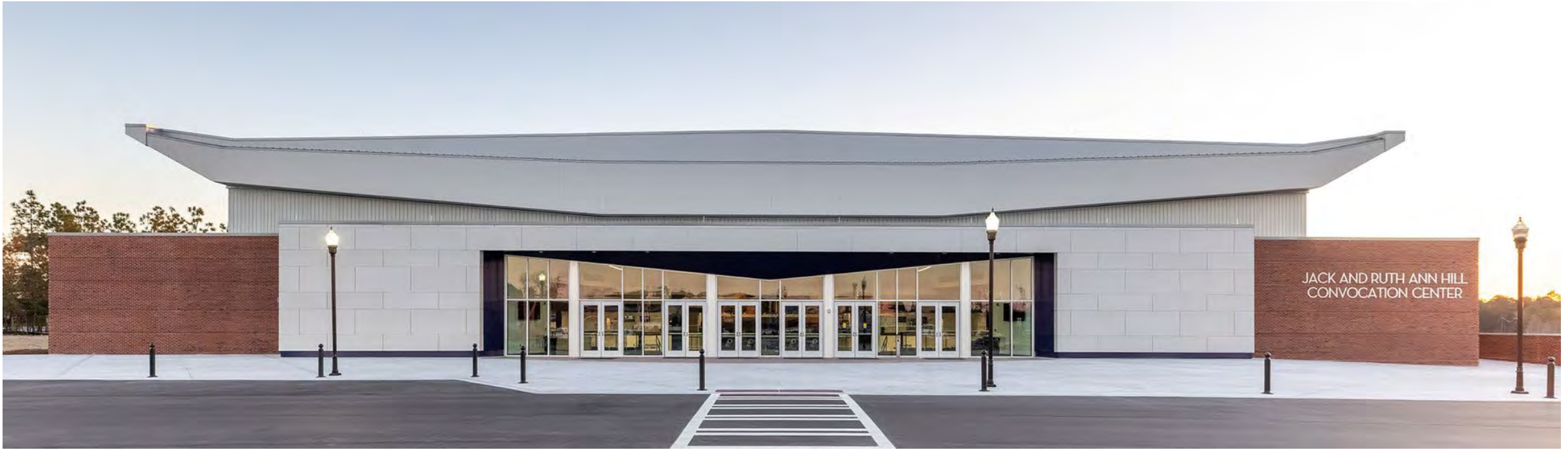
Jack and Ruth Ann Hill Convocation Center, Georgia Southern University, Statesboro, GA Size: 95,000 SF, 19 Acres Construction Cost: $64.4M Role: Civil engineering Sub to AECOM/LS3P
