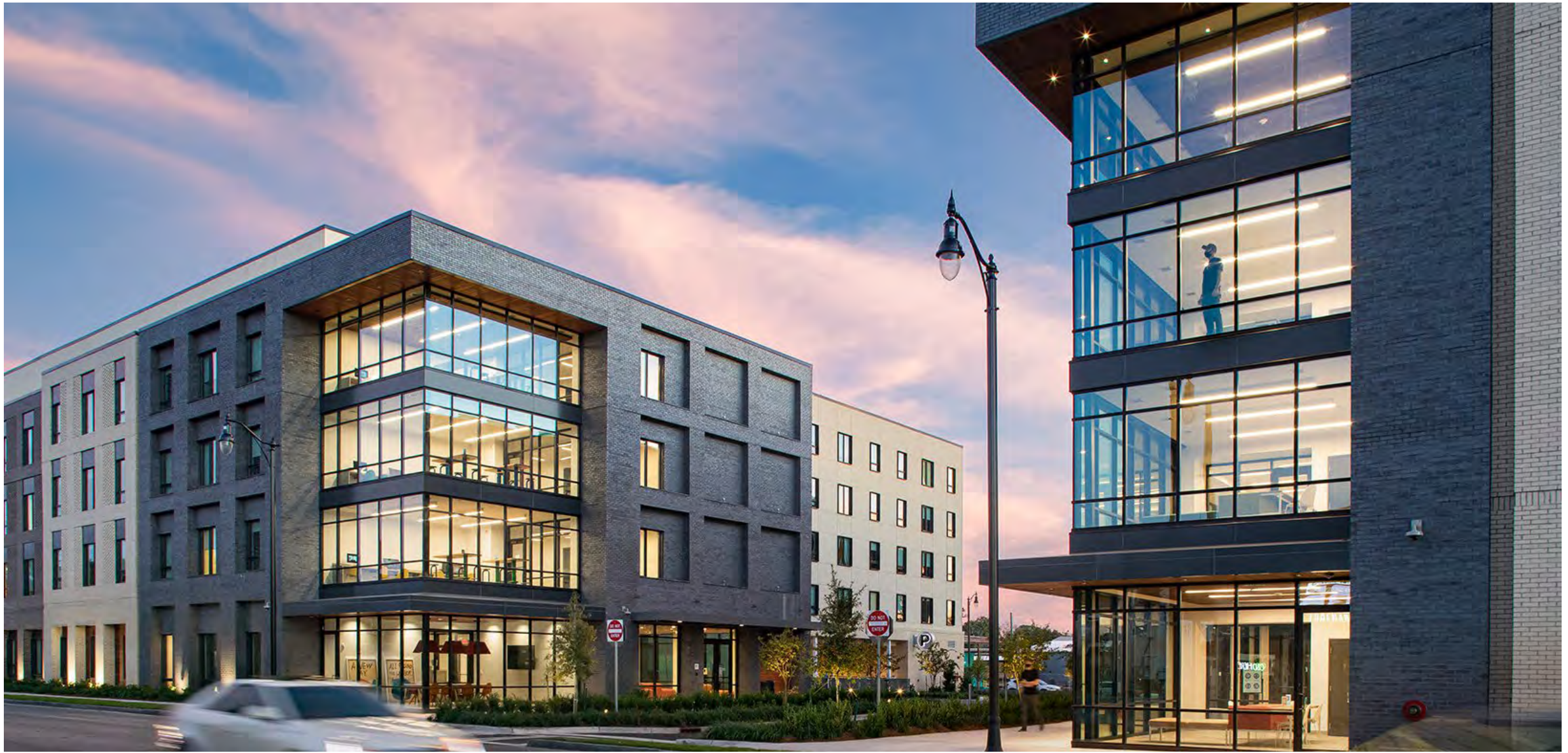
Victory Village, Savannah College of Art and Design, Savannah, GA Size: 250,000 SF Role: Civil engineering Construction Cost: $54M
