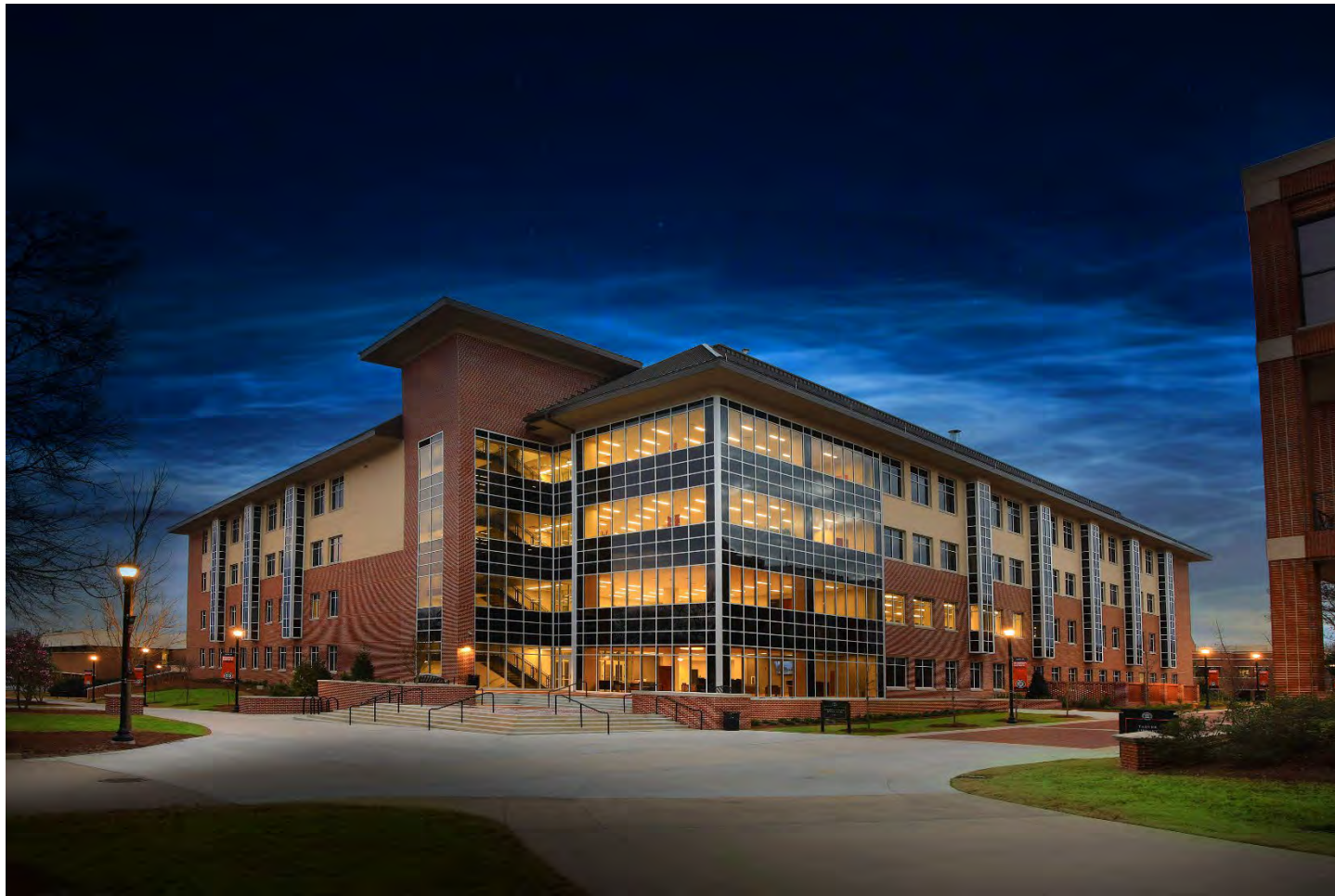
Spearman C. Godsey Science Center, Mercer University, Macon, GA Size: 144,000 SF Role: Architecture, civil + structural engineering Construction Cost: $44M
