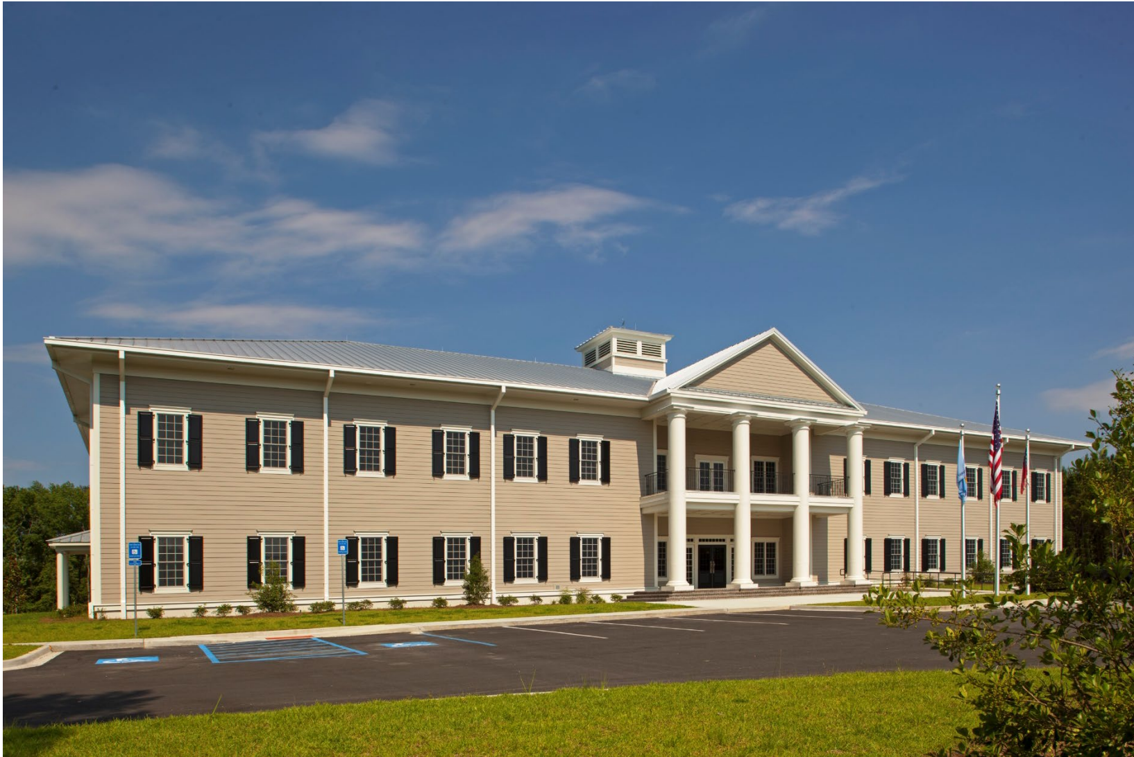
Bryan County Administrative Complex Bryan County, GA Size: 30,000 SF Role: Lead architect/engineer
