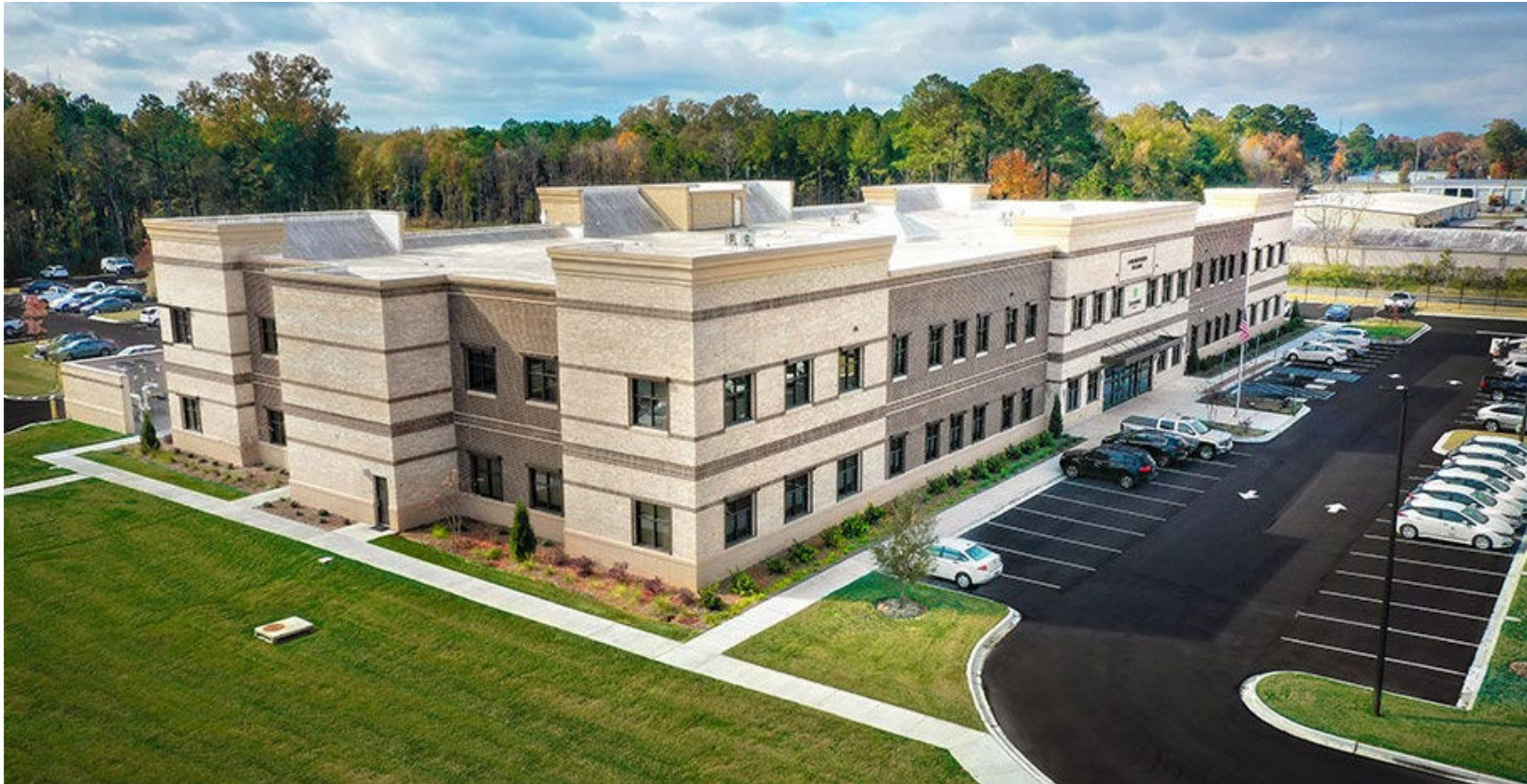
Floyd Adams Jr. City Services Complex Savannah, GA Size: 124,000 SF Role: Lead architect/engineer
