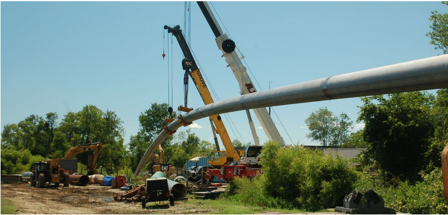
Ashley River Crossing 36" Water Transmission Main Charleston, SC Completion Date: 2018 Size: 4,700 LF of 36-inch steel waterline installed via HDD
