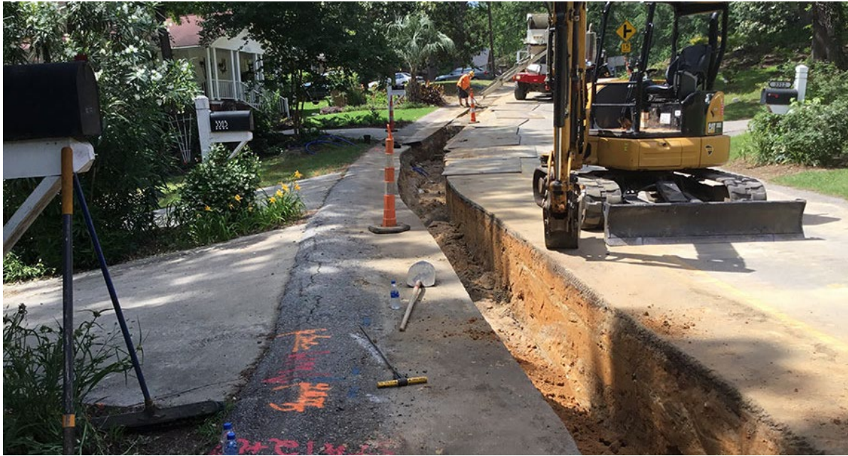
Earlewood Neighborhood Water Quality Improvements Columbia, SC Completion Date: 2020 Size: 27,600 LF
