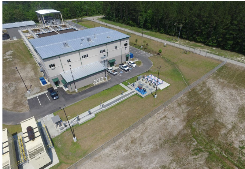
City of Richmond Hill Sterling Creek 4.0 MGD WWTP Richmond Hill, GA Completion Date: 2016 Size: 4.0 MGD flat plate membrane BNR plant
