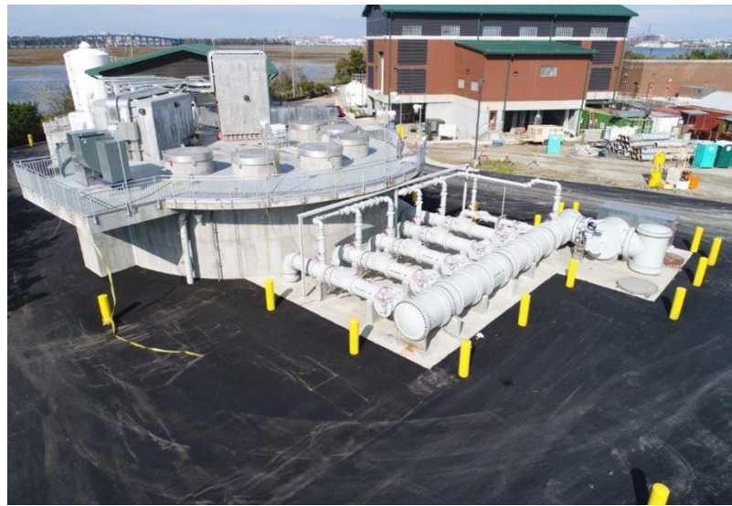
Phase V West Ashley Sewer Tunnel & Influent Pump Station Charleston, SC Completion Date: 2022 Size: 120-foot-deep, 1.6-mile-long tunnel and new 60 MGD influent pump station
