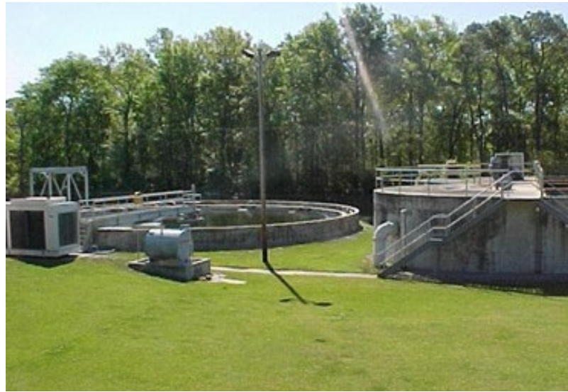
Georgetown Water Reclamation Facility Savannah, GA Completion Date: 1972-2004 (original + multiple expansions) Size: 2.45 MGD oxidation ditch type
