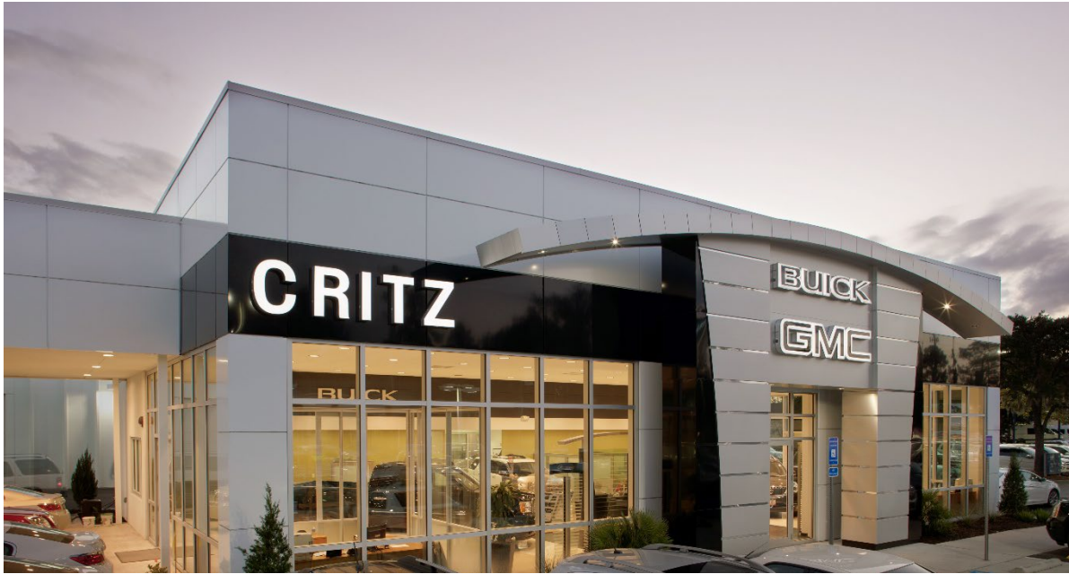
Critz Buick-GMC Dealership Savannah, GA Size: 4,500 SF Role: Architect & Engineer of Record
