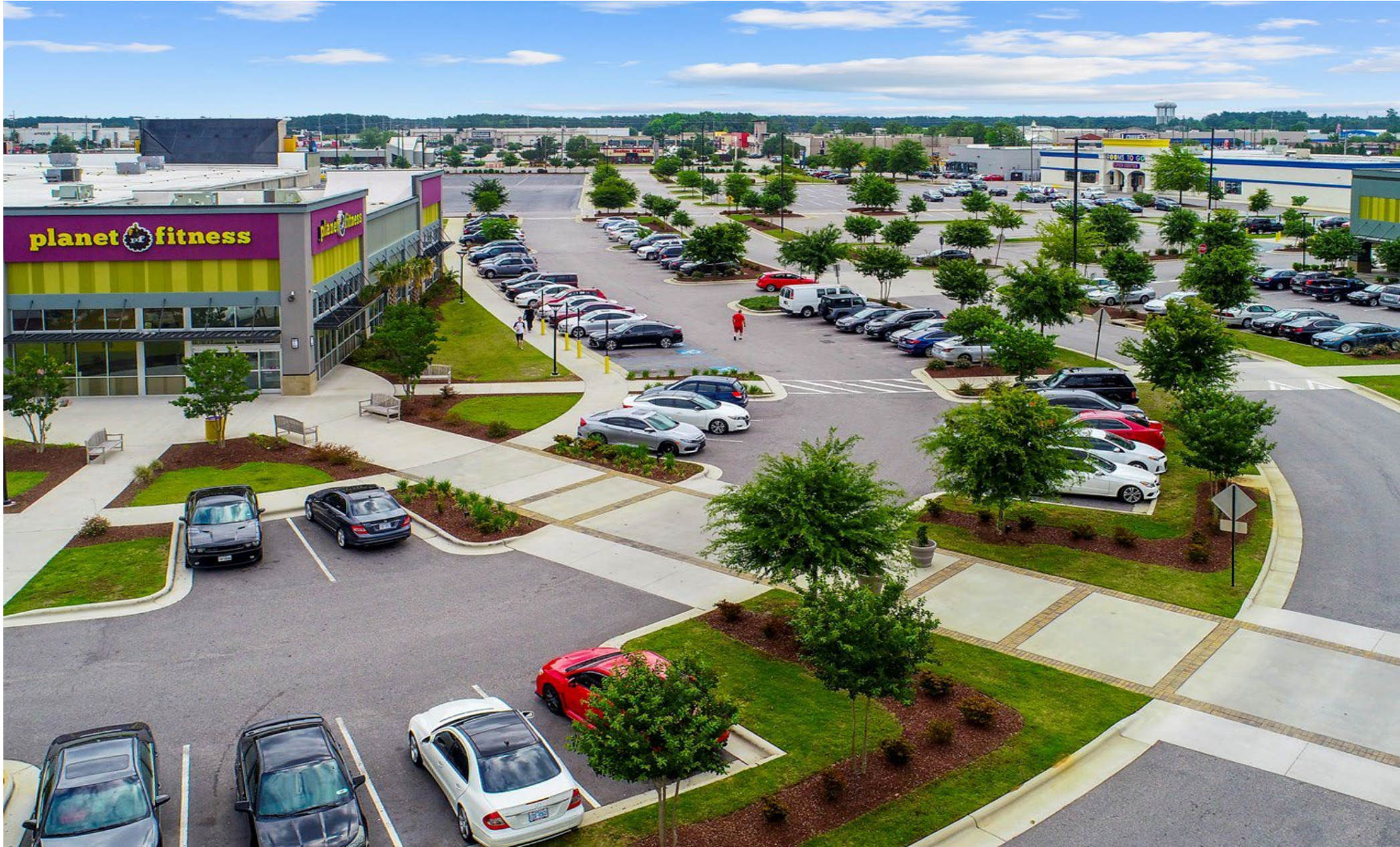
Marketfair Mall Fayetteville, NC Role: Civil Engineering & Site Development
